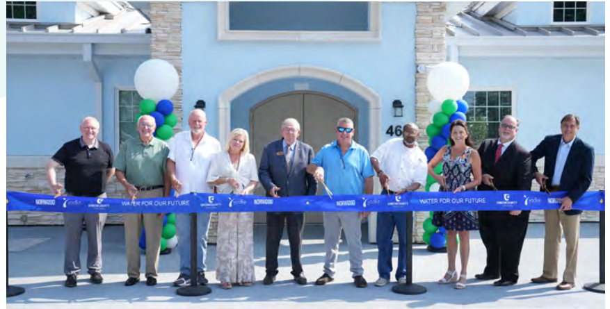
Water intake facility and pump station ribbon-cutting ceremony in Norwood. (Pictured from left to right: Norwood Town Administrator Ray Allen, Norwood Commissioner Wes Hartsell, Norwood Commissioner Keith Morgan, Norwood Mayor Linda Campbell, Union County Commissioner Richard Helms, Norwood Commissioner Robbie Cohen, Norwood Commissioner James Lilly, Union County Board of Commissioners Vice Chair Melissa Merrell, Union County Commissioner David Williams, and Union County Manager Brian Matthews.)
